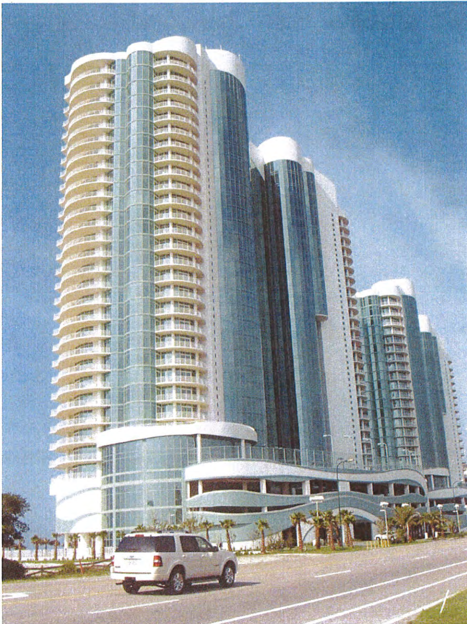
LOOKING WEST AT PROJECT (05/21/10)
