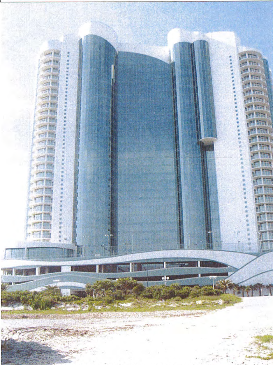
LOOKING SOUTH (FROM NORTH SIDE) AT PROJECT (05/21/10)
